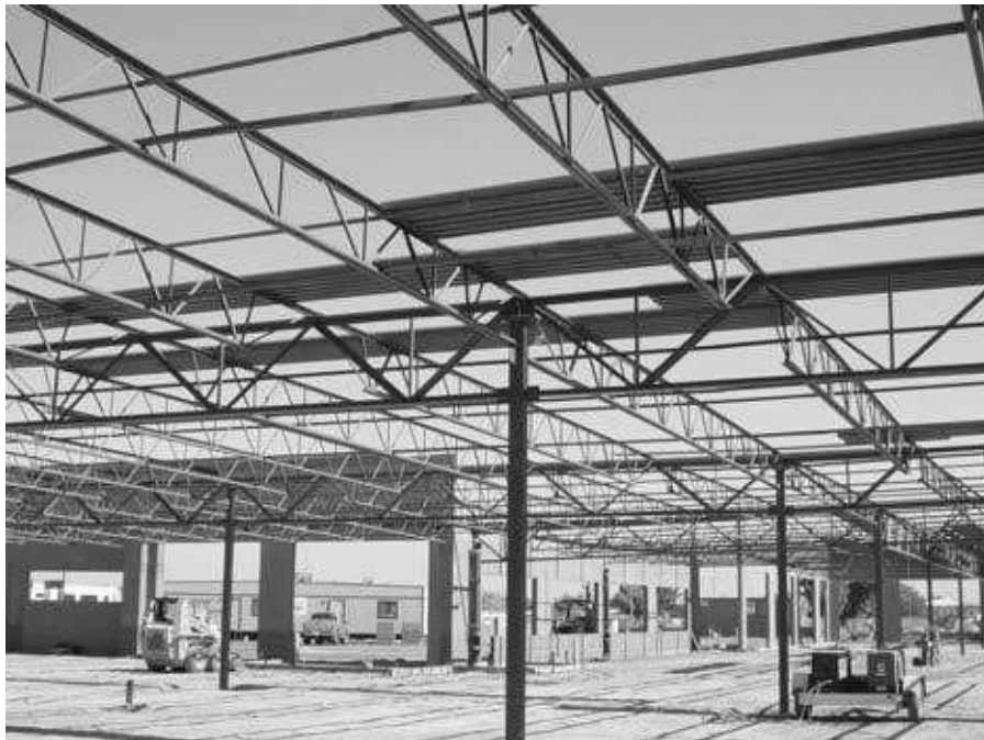
Truss made of structural steel for the structural support of a building.
