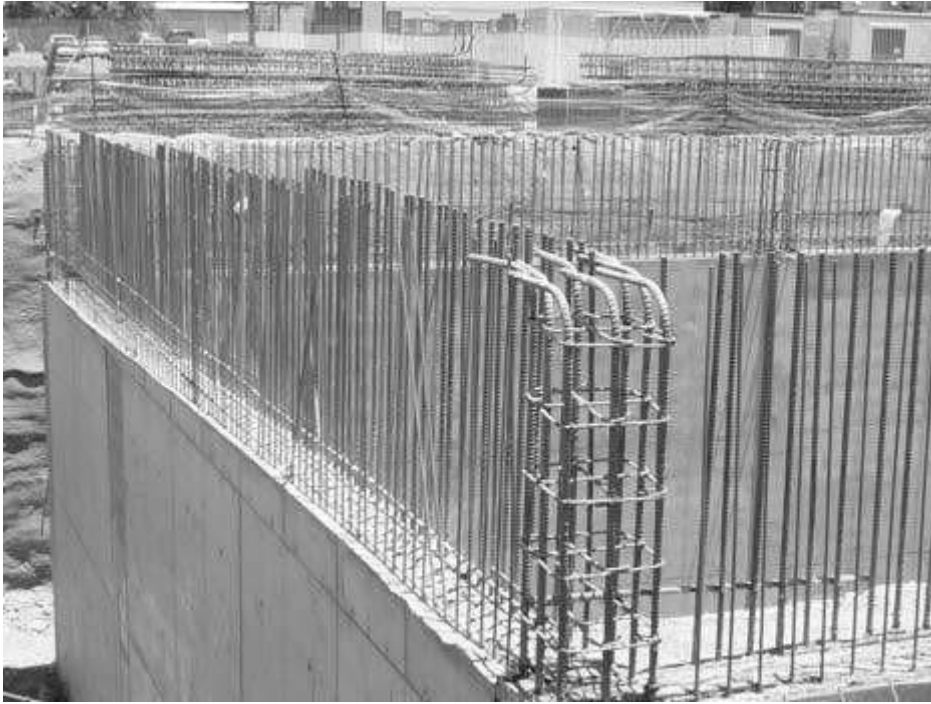
Steel rebars used to reinforce portland cement concrete wall.
